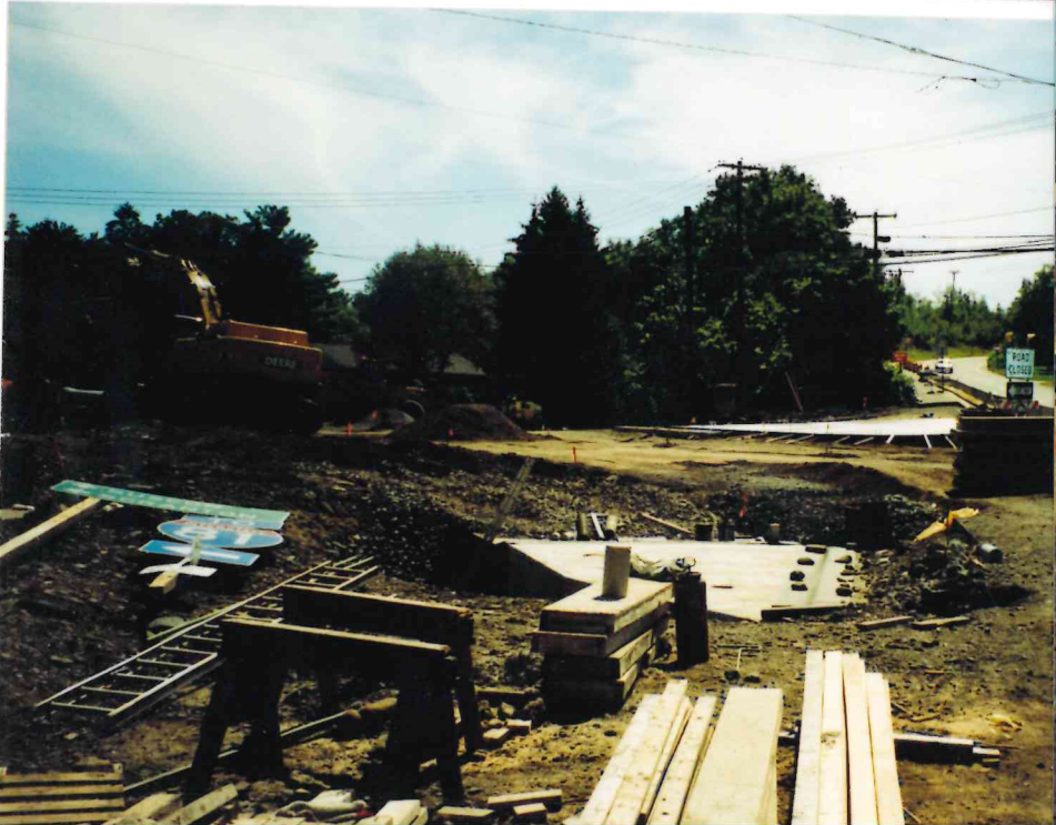
BEAR CREEK ROAD CHESTNUT STREET INTERSECTION RECONSTRUCTION/ TRAFFIC SIGNAL UPGRADE
